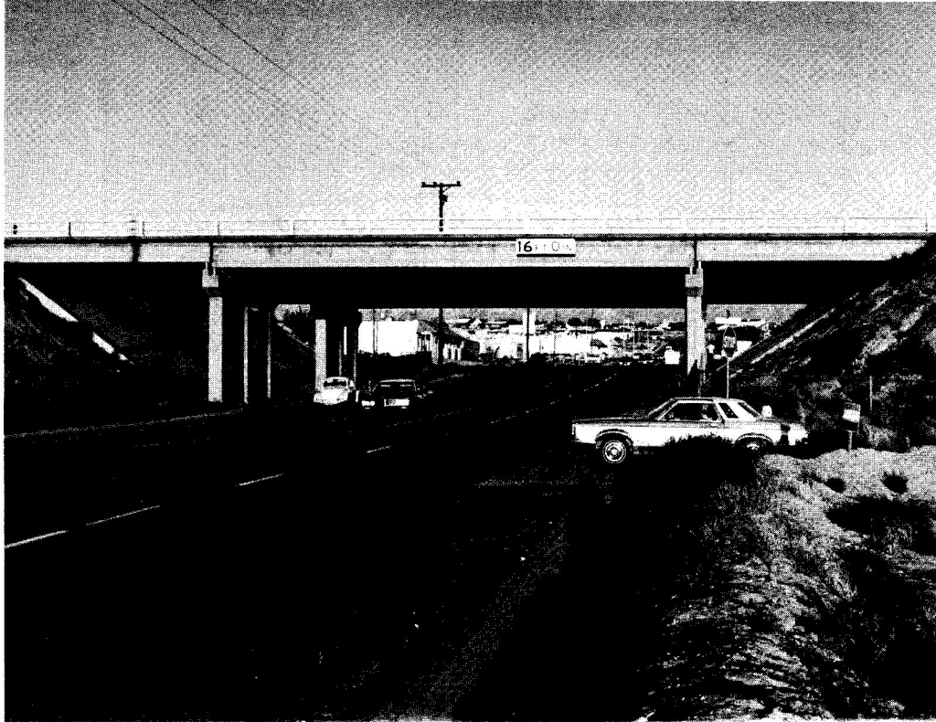
Figure 1 Southbound bridge crossing Missouri Street on I-25 in Las Cruces, New Mexico.
